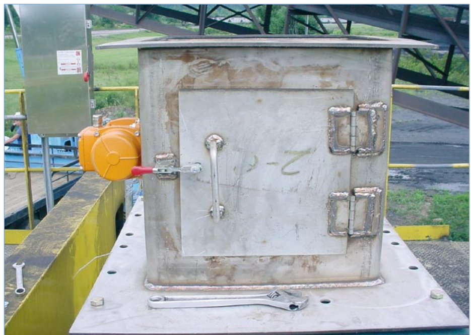
Figure 5. Stainless crusher feed chute with inspection door, vibrator and local motor lock out panel.
