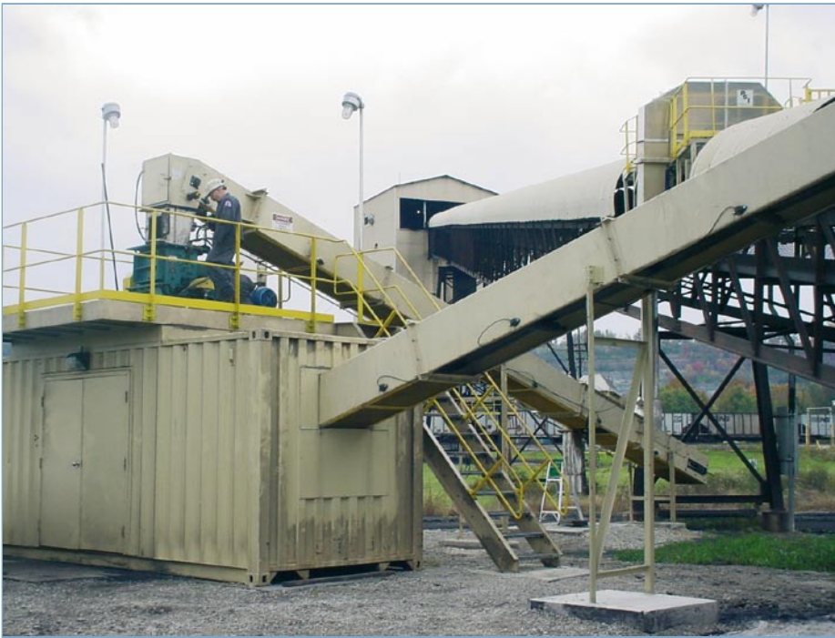
Figure 6. Compact modern cross-belt mechanical sampling system.
